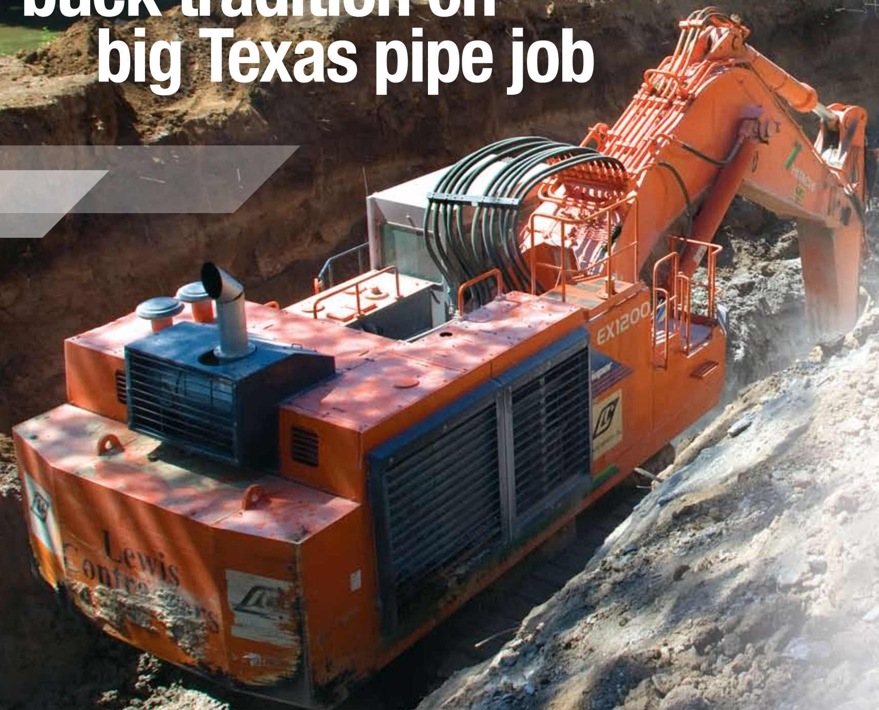
Two EX1200 Excavators, equipped with Leading Edge rock buckets, make the final trench to grade through blue limestone and dirt on the South Fork San Gabriel Interceptor project near Georgetown, Texas.
